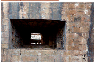
Figure 3. 1 Francisco of Holland. Drawing of the fortress of San Sebastián. The graded cannon embrasures level is highlighted and in close-up. 2. Graded cannon embrasures at the Fuenterrabía fort
